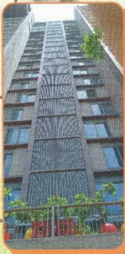
Bird Net Installation on Building Duct
